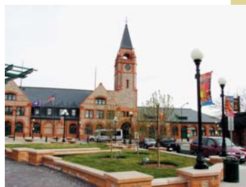
The Old Train Depot
